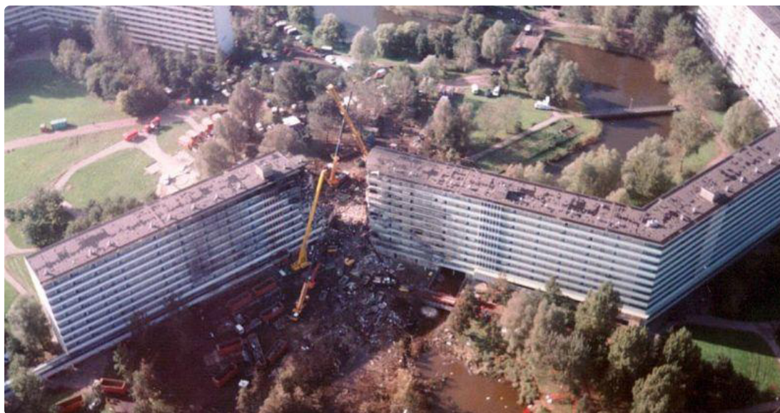
▼ Figure 1. Photograph taken after the disaster showing the damage of the Boeing 747 crash.
